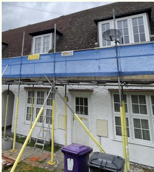
Figure 4 shows three inspection stages during the materials' application. Top is after the original render's removal, middle is after one coat of Diathonite, and bottom is the final finish. Source: Wates and Ambue.
