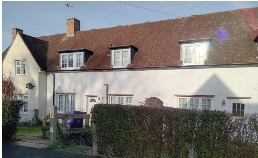
Figure 2 shows the property before works (above) and after (below). Source: Wates.
