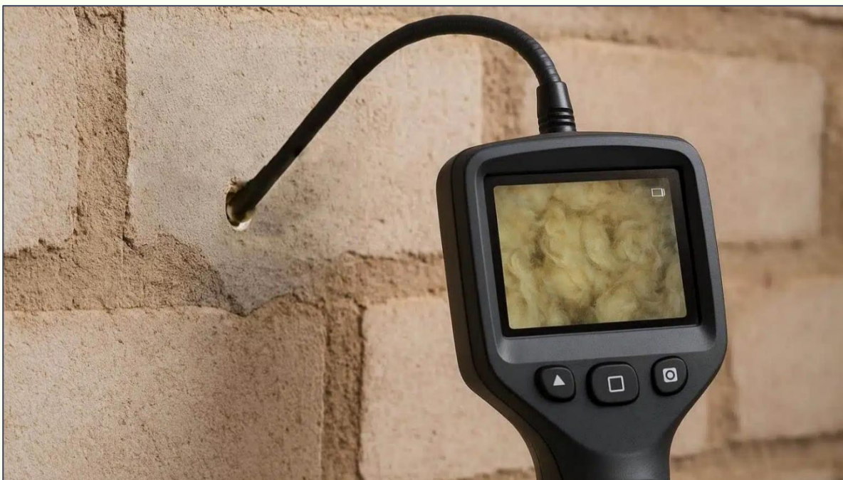
Figure 2. Borescope inspection carried out by Harpr Surveyors
