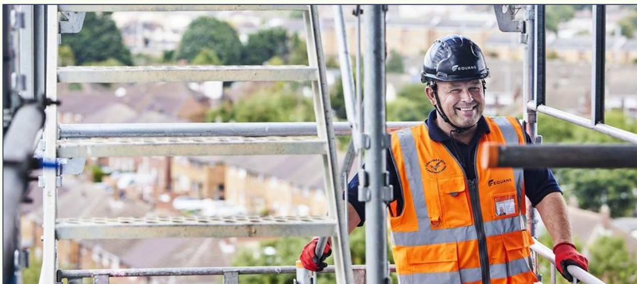
Figure 1. Equans employee delivering cavity wall insulation extraction
