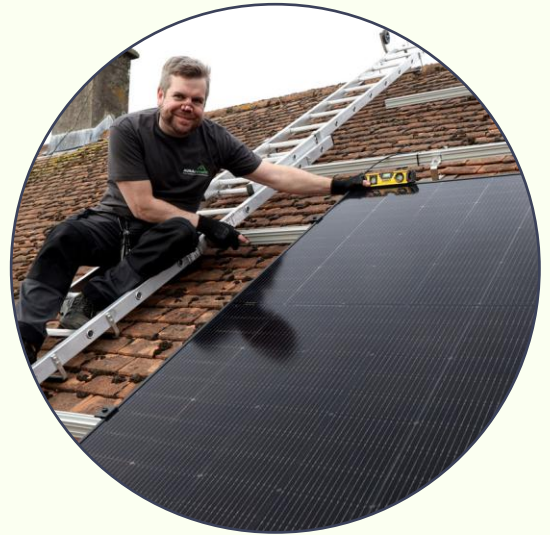
Figure 2 Aura Retrofit Contractor fitting Solar
