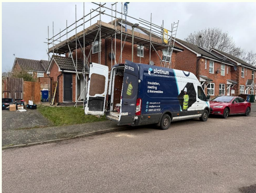
Figure 3: Installation of measures to Pauline's home (Source: OCC)
